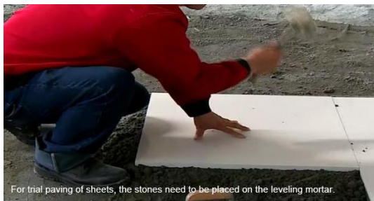
For trial paving of sheets, the stones need to be placed on the leveling mortar.
